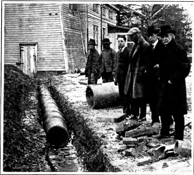
LAYING A ROGERS UNDERGROUND ANTENNA
